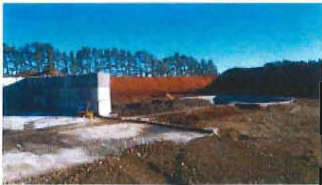
Figure 4 Reception area and mixing bay (left), with drain and sump (right)
