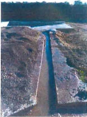
Figure 5 Drain from reception area and mixing bay to the sump
