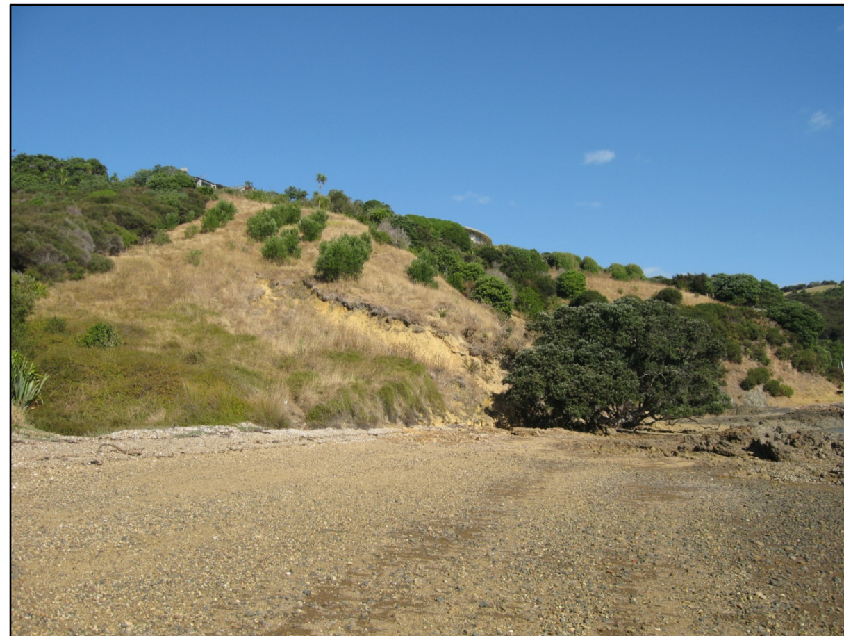
View of Slip on Reserve – Date: 27-02-2013 – Low Tide
